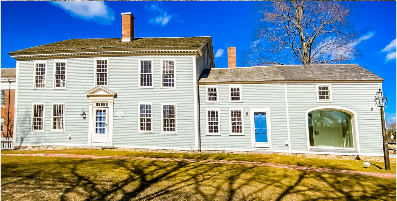
The Loring Parsonage, Home of the Sudbury History Center and Museum Pictured at top, circa 1930, and with recent renovations at bottom in 2020
